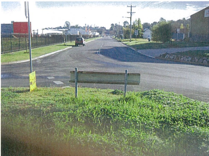
Figure 4 Schubach St to north
