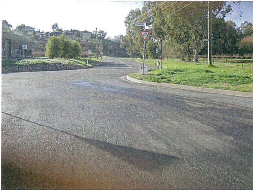
Figure 3 Intersection to East
